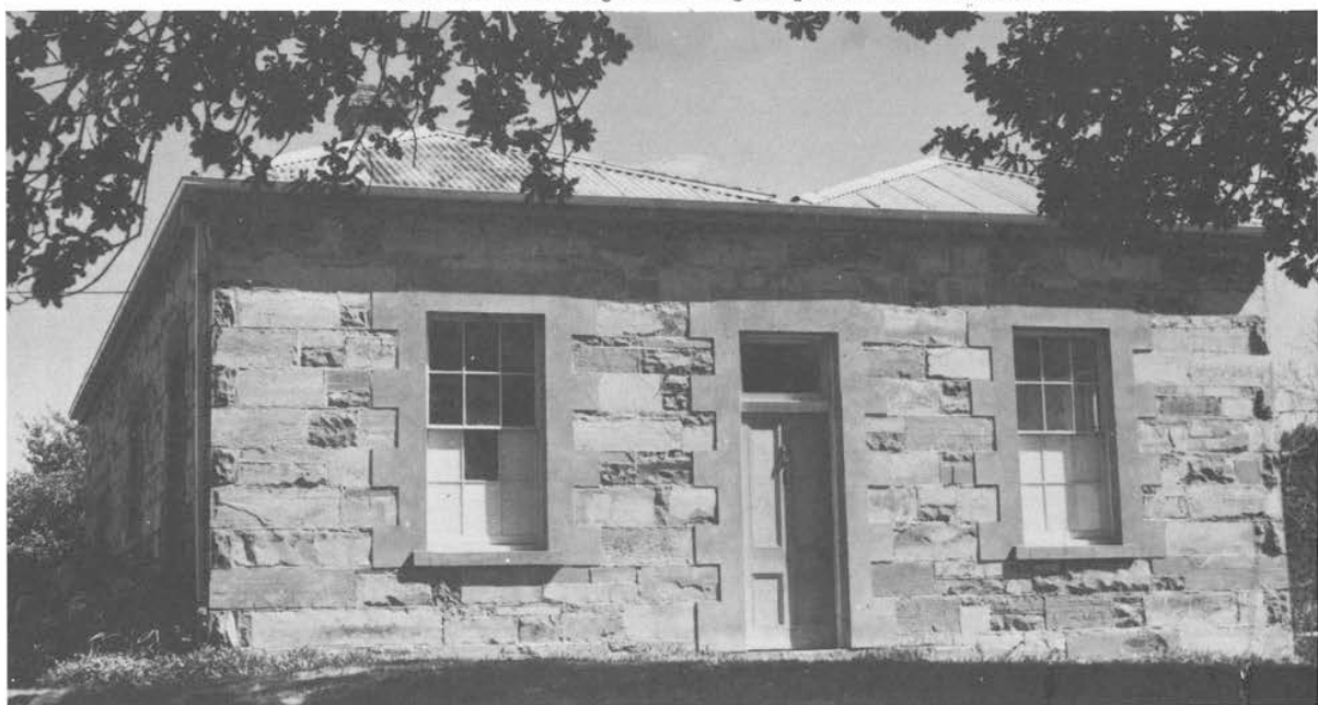
Von Schramm's cottage in its original position in Doncaster Road
